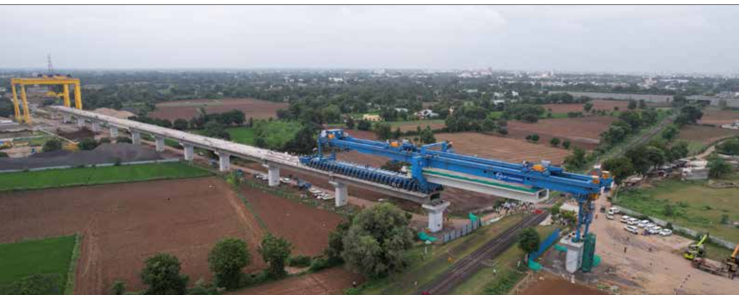
Indigenously designed and manufactured Full Span Launching Machines for Mumbai-Ahmedabad High-Speed Rail (MAHSR)
