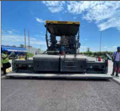
CCPR implementation at Meerut-Aligarh-Ghaziabad road project
